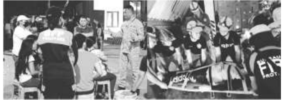
BFP CENTRAL LUZON RESCUERS SEARCHES FOR TRAPPED VICTIMS FROM A COLLAPSED BUILDING IN MEYCAUAYAN – Bureau of Fire Protection Central Luzon (BFP-CL) Director C. Supt. Roderick P. Aguto (left photo, right) is personally getting important information from the employees of E-One Consumer Trading Corporation located at Silver Street, Muralla Industrial Park in Meycauayan, Bulacan, which the second floor of its building collapsed and trapped four employees under the rubble. Right photo shows BFP-CL Special Rescue Force team led by Sr. Supt. Ronnie B. Barrera rushing one of the victims to the waiting ambulance to be brought to the nearest hospital for immediate treatment. BFP Bulacan Provincial Director Supt. Vilma R. Tuscano and Meycauayan City Fire Director C. Insp. Antonio De Jesus, Jr. also rushed to the scene to help lead the rescue operation. Three workers died in the incident. (Benjie J. Murillo / BFP-CL Photos)
