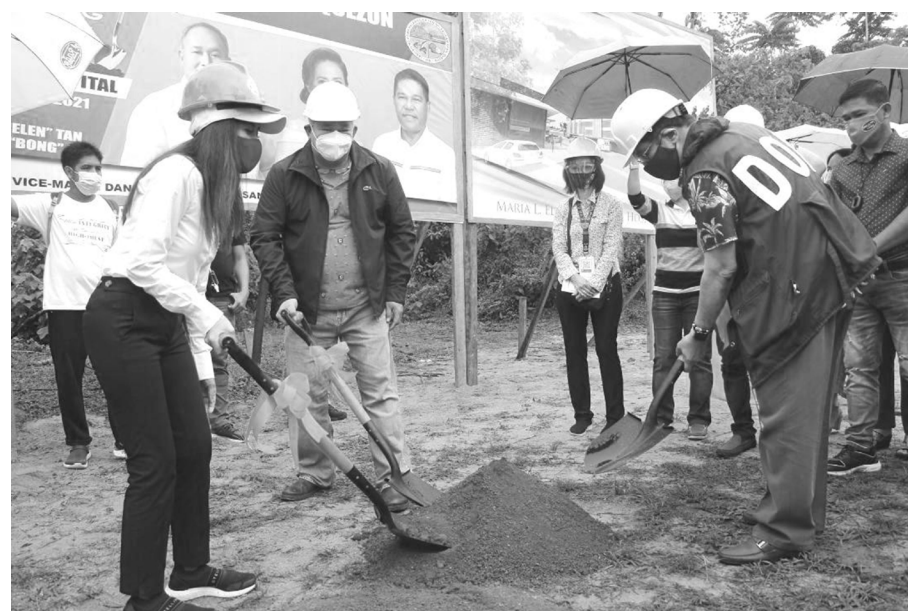
(R-L) DOH-CALABARZON Eduardo C. Janairo together with 4th District Representative Heolen Tan and Tagkawayan Mayor Carlo Eleazar leads the groundbreaking ceremony for the proposed three new buildings for the Maria L. Eleazar General Hospital in Tagkawayan, Quezon on January 14, 2021
