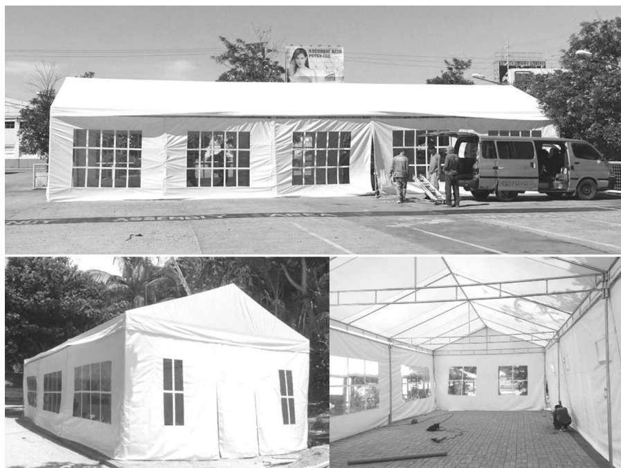
The 44-bed capacity heavy duty collapsible modular tent which will serve as emergency intensive care unit and ward for Covid patients in CALABARZON. It is a close tent with a 5-meter wide and 12-meter-long floor area fully covered with soft PVC side wall and with eave height. One modular tent cost Php294,850.00
