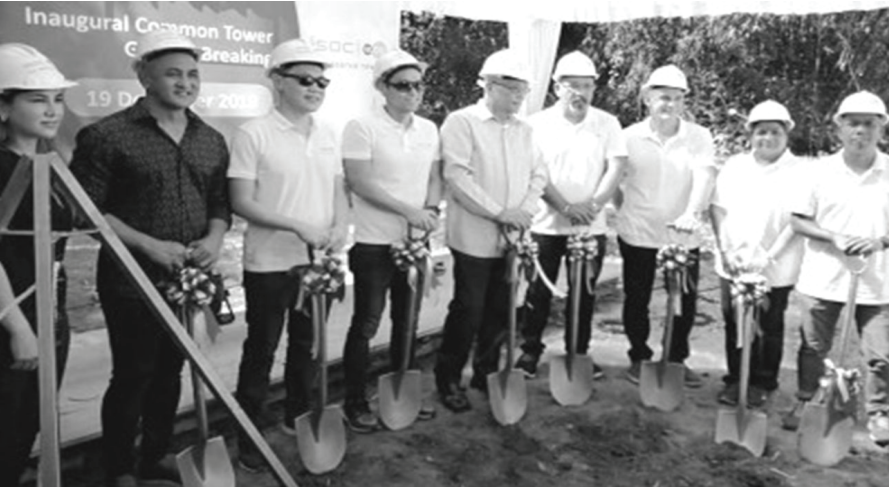
COMMON TOWER. Department of Information and Communications Technology (DICT) Undersecretary Elizeo Rio (leftmost), with edotco and ISOC infrastructure officials, led the groundbreaking rites for the construction of the first common tower in Addas Greenfield Village, Bacoor City, Cavite on Thursday (Dec. 19, 2019). The infrastructure aims to reduce the country's subscriber-to-tower ratio which currently stands at over 7,000 subscribers per tower. (PNA)
