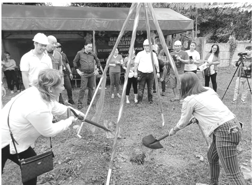
Groundbreaking by CJ5 Morning Sun Holdings Corporation represented by Ms. Ma. Theresa Puno (left) and Lotus Group of Companies represented by Leasing Officer Ms. Jazel Gomez Loyola of the soon to rise "EPI CENTER LEIZURE ENTERTAINMENT PLAZA" which shall be built along Diversion Rd. Palico IV Imus City fronting the Medical Center of Imus City. With related story at my column. (Sonny B. Anarna)
